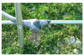
If the shelter is to be used for livestock housing, it is necessary to secure the anchoring bolt joint against abrasion with fabric and adhesive tape. **16.** Lay the main tarpaulin along the long side of the shelter. Pull the tarpaulin over the structure using the supplied tensioning ropes.
