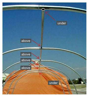
9. Place the structure in the desired location and measure the diagonals of the shelter floor from one corner tube to the other as shown in the picture.
