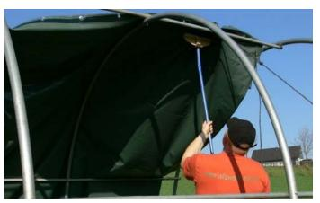
The correct position of the tarpaulin is reached when the welded-on 10 cm wide strip (reinforcement) is located exactly over the top connecting pipe.
